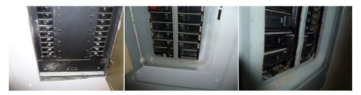
The below pictures are of unsecured disconnects. These are so common. Secure all disconnects as well as any other electrical device box. Zip ties suffice.
