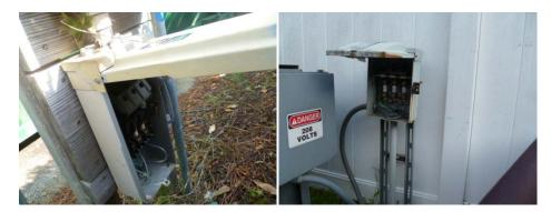
The timer and panel boxes below are missing their internal covers. Always secure the timer boxes with zip ties even if the factory plastic cover is in place as they can easily fall out. As for a missing cover on a panel box...find it and put it back on.
