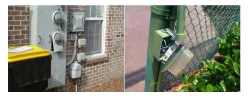
The below electrical hazards are all too common. The space between the breakers and the cover, or the space between the panel's interior cover and external ones causes a health and safety deficiency when the gap is more than ¼".
